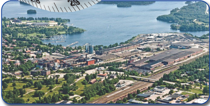
Key Client: Turner & Coates has been working with Swedish steel manufacturer Ovako, since 2013.
